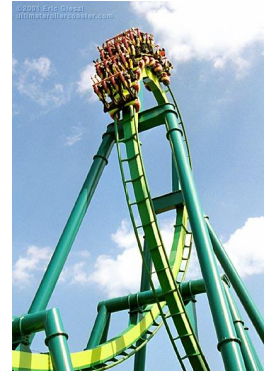
Clothoid loop illustrated by the roller coaster the Raptor located at Cedar Point.
