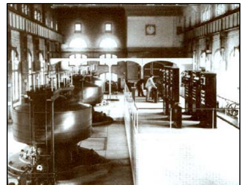
The inside of the first AC Power Plant, the Adam's power station. Built November 16, 1896 at Niagara Falls.
