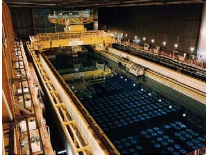
Figure 6. Nuclear waste containers are stored in cooling pools to contain radiation.
